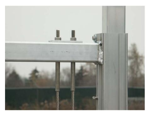
9: Slide Tube Connector onto Corner Post D. Tighten with the  $3/8 \times .75$ " screws, washers and square nuts as shown.
