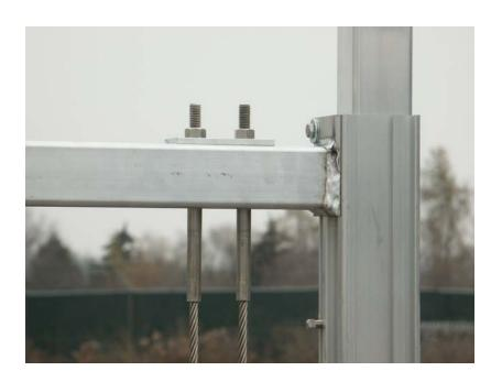
18: Attach the 5/16 carriage bolt, washer, and nut to the lower cable angles. Repeat this for all (4) angles.
